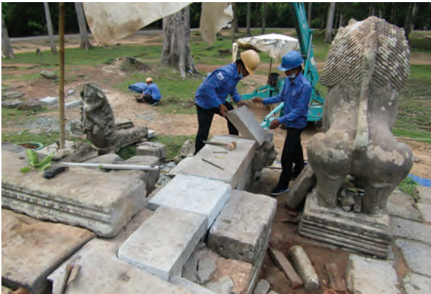
Fig.5.25, 5.26 Large scale platform improvement was implemented. Laterite and Sandstone were inserted under the Balustrade.
