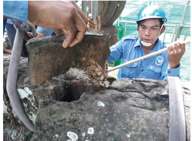
Fig.5.35 Remove of deteriorated mortal of Naga
