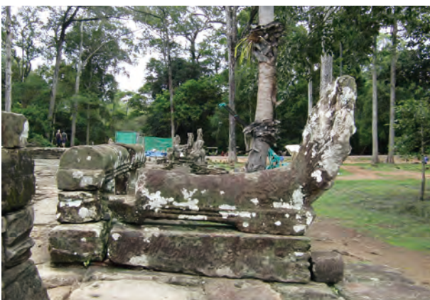
Fig.5.21, 5.22 Before and After restoration, Newsandstone bansement was inserted instead of substitute element/ 71.2.1
