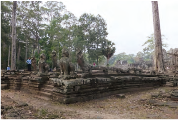
Fig.5.15 Before restoration at Northeast part of C71.1-1 .Platform was heavily distorted.
