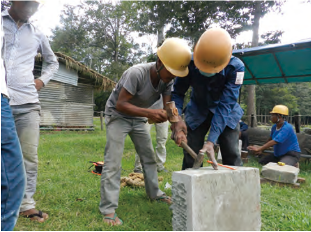
Fig.5.2 Onsite job training for stone processing
