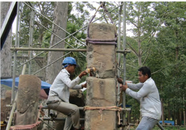
Fig.5.50 [T69.2] Repairing of Basement of Bulastrade
