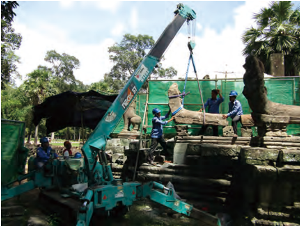
Fig.5.34 Reconstruction of balustade/T67.2.
