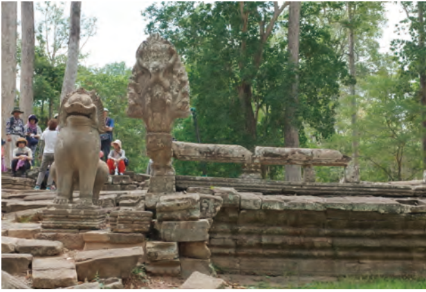
Fig.5.23, 5.24 More than 60cm subsidence at southeast gate of causeway(71.2-1). Naga and Lion statues are at danger of collapse.
