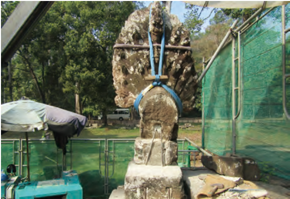
Fig.5.36, 37 Before restoration, the Naga statue at T65.3 had no trunk and couldn't stand without many iron pin inserted in previous restoration. However, we could found piece of trunk from scatter stone near this area, so that this statue could stand without support oafter restoration.
