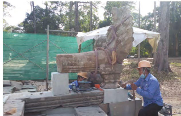
Fig.5.27, 5.28 After improvement of platform, Naga Balustrade were reconstructed. New sandstone was added for Post and Basement in need.
