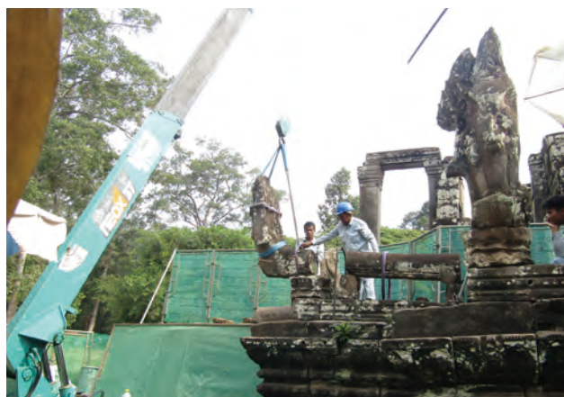
Fig.5.41 [T61.3] Dismantling of Naga Statue
