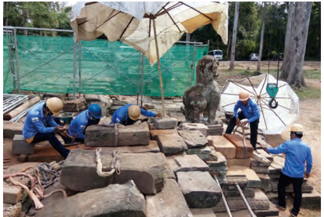
Fig.5.25, 5.26 Large scale platform improvement was implemented. Laterite and Sandstone were inserted under the Balustrade.
