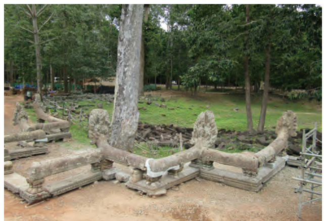
Fig.5.51 [T69.2] Trial Assembling of Balustrade on the ground
