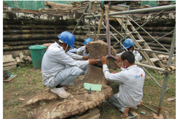
Fig.5.36, 37 Before restoration, the Naga statue at T65.3 had no trunk and couldn't stand without many iron pin inserted in previous restoration. However, we could found piece of trunk from scatter stone near this area, so that this statue could stand without support oafter restoration.
