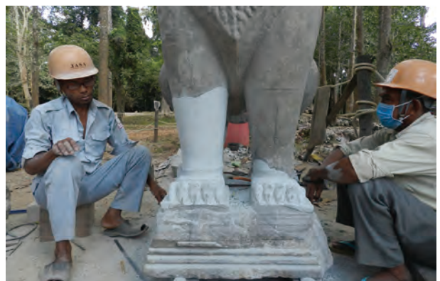
Fig.5.29, 5.30 Due to the deterioration of the concrete material from the previous restoration and the danger of collapse, the lion's four legs were replaced with new sandstone.C71.1-1(71.1.1.9.1.4)
