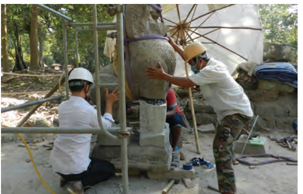
Fig.5.29, 5.30 Due to the deterioration of the concrete material from the previous restoration and the danger of collapse, the lion's four legs were replaced with new sandstone.C71.1-1(71.1.1.9.1.4)
