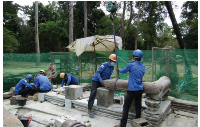
Fig.5.20 Reconstruction work, adjusting post height/ C71.2-1 east part
