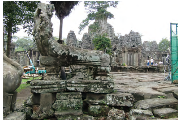
Fig.5.23, 5.24 More than 60cm subsidence at southeast gate of causeway(71.2-1). Naga and Lion statues are at danger of collapse.
