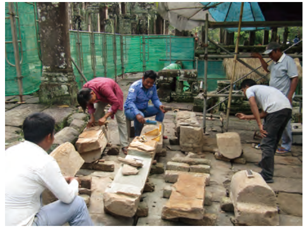
Fig. 5.70 Repair of excavated balustrade elements
