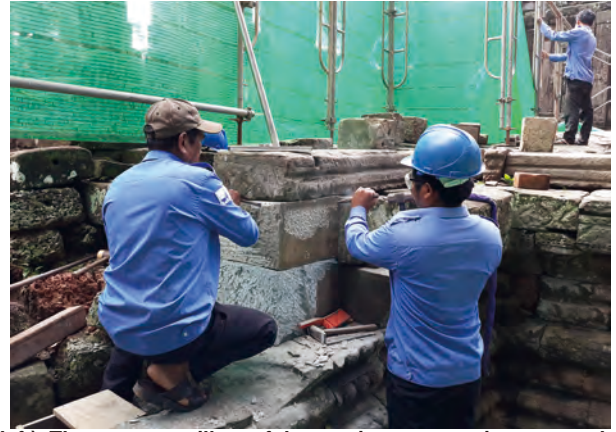
Fig.5.32, 5.33 Discussion with JASA experts on restoration methods(left). The concrete pillars of the previous restoration were to be removed and new sandstone material was to be inserted into the platform(right)/T67.2.
