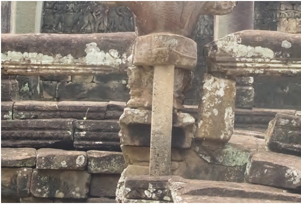
Fig.2.1 Concrete support under Naga
