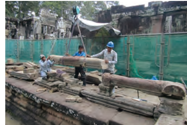
Fig. 5.74 Reconstruction of Balustrade
