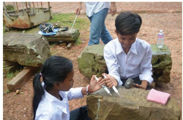
Fig.6.9, 10 Sudents received instruction from JST technical staff and had hands-on experience cleaning the stone using a brush, injecting reinforcement material using a syringe, and processing new sandstone using a chisel
