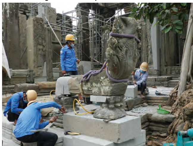
Fig.5.12 C71.3.2: New Sandstone Supply for Naga
