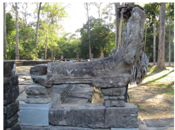
Fig.5.21, 5.22 Before and After restoration, Newsandstone bansement was inserted instead of substitute element/ 71.2.1
