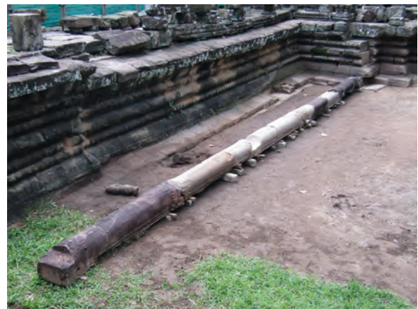
Fig. 5.65(left), 5.66(right) Trial Assembling work on the ground including found elements
