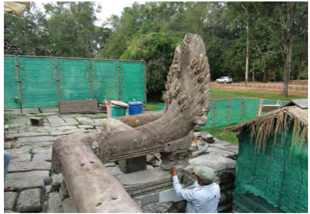
Fig.5.44, 45 [T62.1] Insert new sandstone block in order to make a level and stable floor surface
