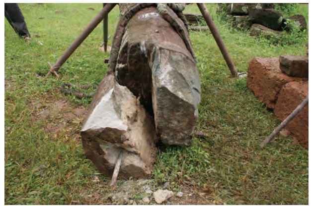
Fig.2.2 Collapsed section due to deterioration of restoration material
