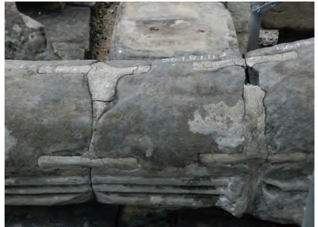
Fig.2.4 Iron pin connection
