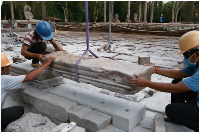
Fig.5.17 Insert new sandstone plate for support under the basement /71.1.1
