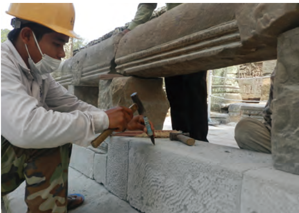
Fig.5.6 T.58.1: New sandstone supply for basement
