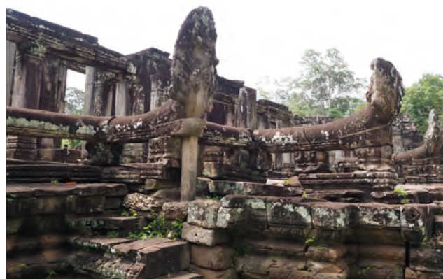
Fig.5.42 [T62.1] Before restoration, Support by concrete pillar was deteriorating.
