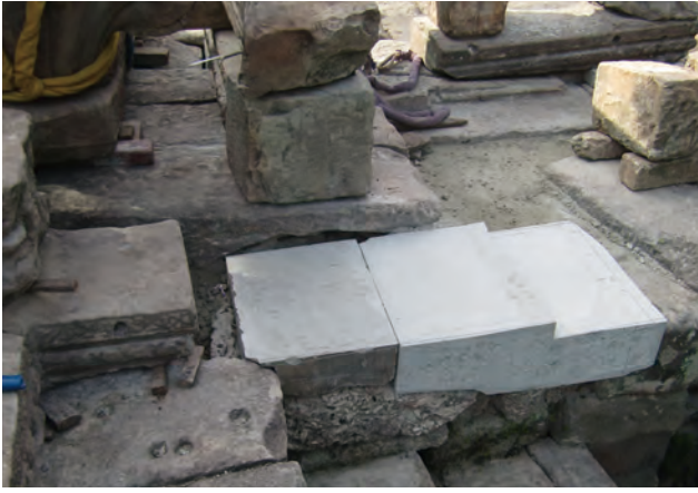
Fig.5.44, 45 [T62.1] Insert new sandstone block in order to make a level and stable floor surface
