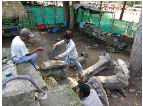
Fig. 5.72 Repair of excavated balustrade elements
