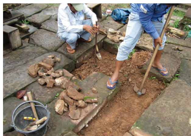
Fig.5.43 [T62.1] Maintenance and improvement of platform floor before install the bulastrades
