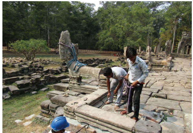
Fig.5.47 [T60.2] Reconstruction of balustrades
