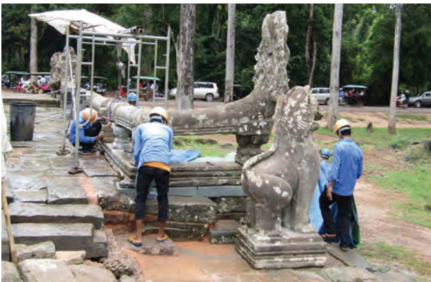
Fig.5.27, 5.28 After improvement of platform, Naga Balustrade were reconstructed. New sandstone was added for Post and Basement in need.
