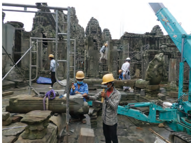
Fig.5.14 C71.4.2: Reconstructing and New sandstone processingWork
