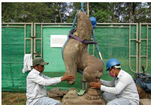
Fig.5.40 [T61.3] Trial Connecting of Lion Statue(61.3.9.1.1)
