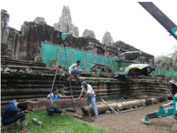
Fig. 5.65(left), 5.66(right) Trial Assembling work on the ground including found elements
