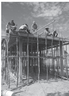
中学校校舎建設中! Junior high school building under construction!
